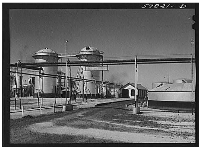
Wolcott, Marion Post. Barnsdall oil refinery. Kansas, 1941.
