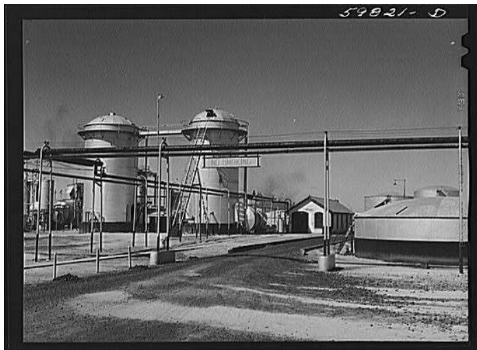
Wolcott, Marion Post. Barnsdall oil refinery. Kansas, 1941.
