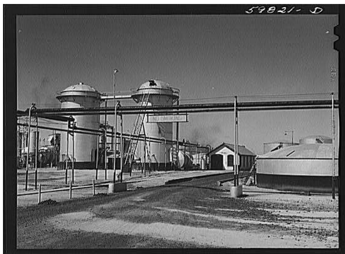
Wolcott, Marion Post. Barnsdall oil refinery. Kansas, 1941.
